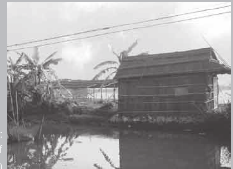
Economics of Architecture : An agrarian cottage made out of tree barks in Zhong Shan
